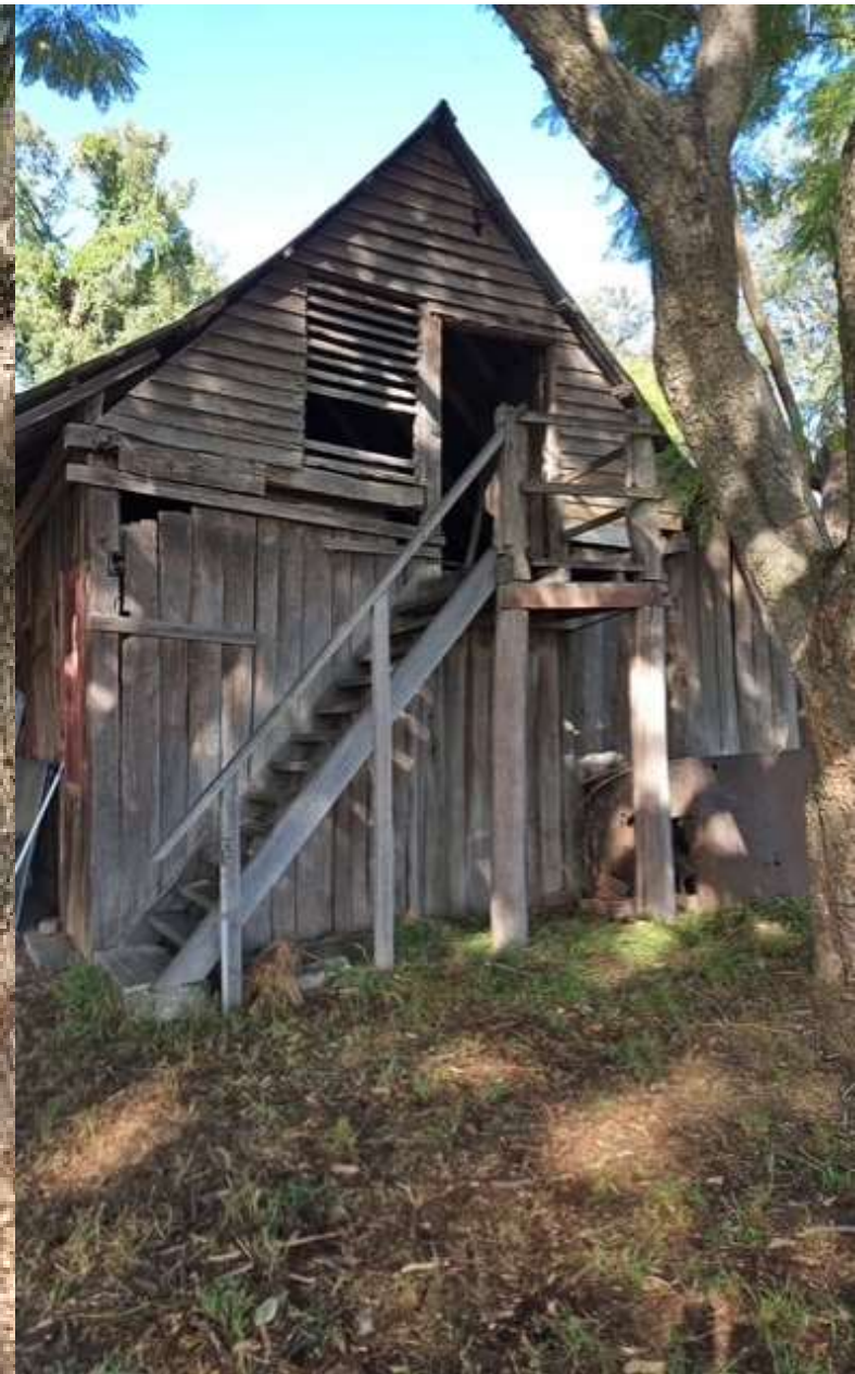
Stable Roof and Cladding Before
