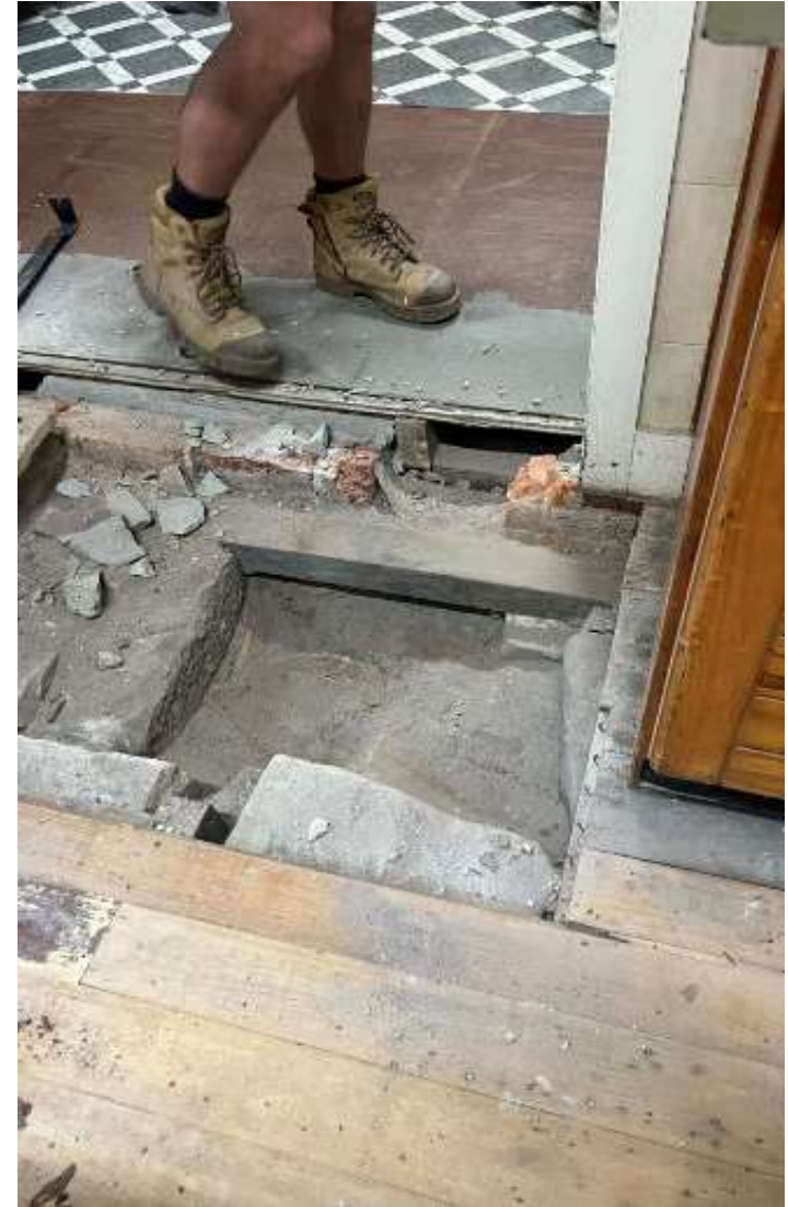
Homestead Kitchen, Laundry flooring and Termite damage before
