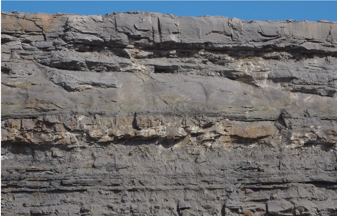
Plate 19: Iron staining due to the partial oxidation of pyrite visible in the lower section of the Archerfield Sandstone.
