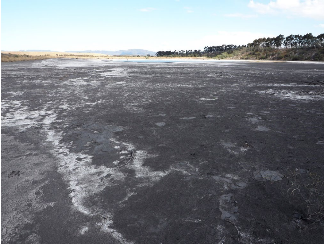
Plate 25: White salts observed across the surface of deposited tailings within the disused Bob's Dump TSF.
