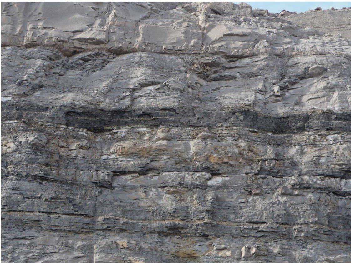
Plate 18: Iron staining and sulphate salts due to the partial oxidation of pyrite associated with the Lemington Seam Group in West Pit.
