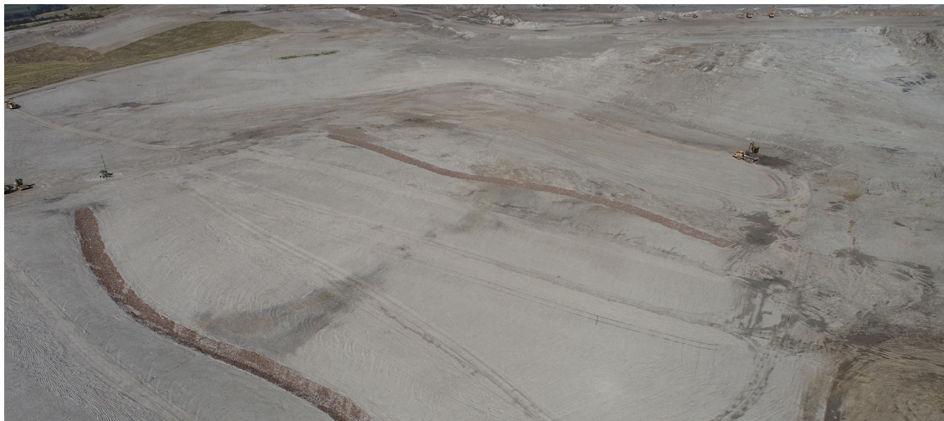
Shaping and rock drain installation at 2025 Cheshunt Rehabilitation
