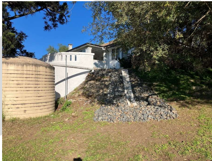
Parapet upgrade and drainage repair
