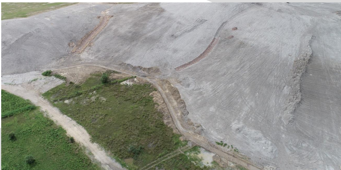
Shaping and Rock Drain Installation at 2025 Cheshunt Rehabilitation
