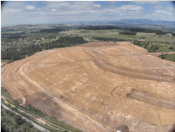
Contour construction and topsoiling at East TSF
