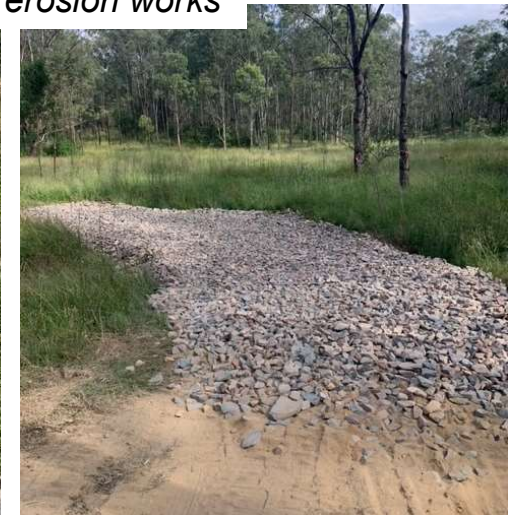
Mitchelhill West offset access track erosion works
