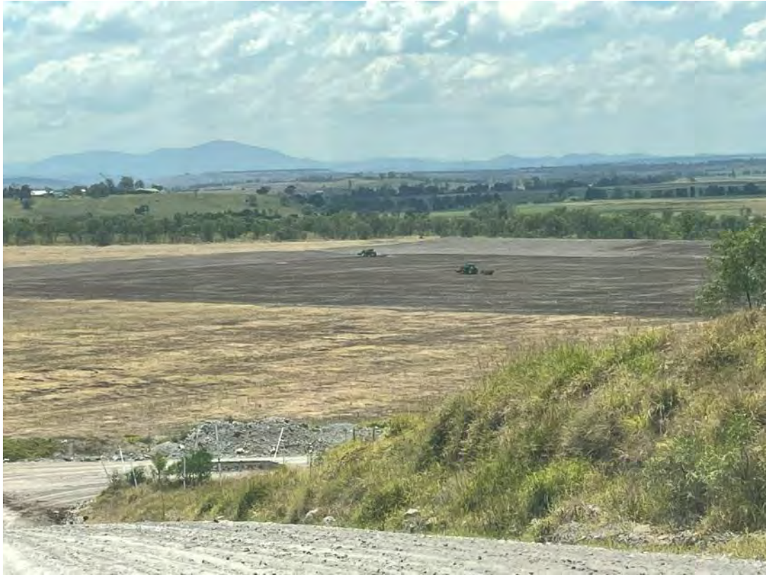
Plate 63 – Active rehabilitation works
