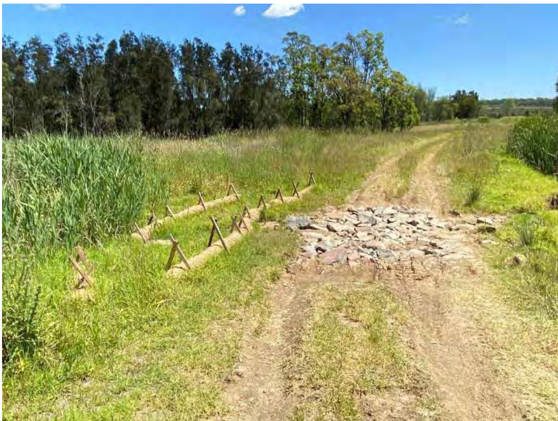
Plate 36 – Sediment control structures observed in place at spill ways
