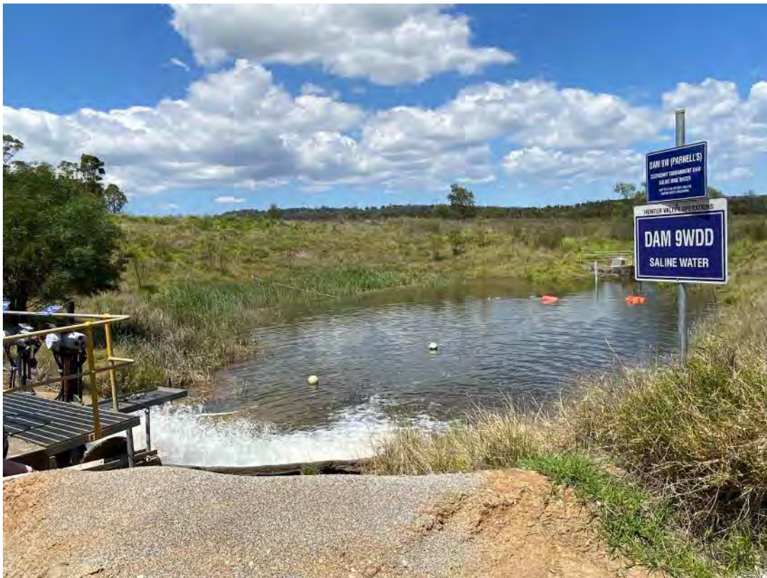
Plate 34 – HRSTS Discharge point Dam 9WDD
