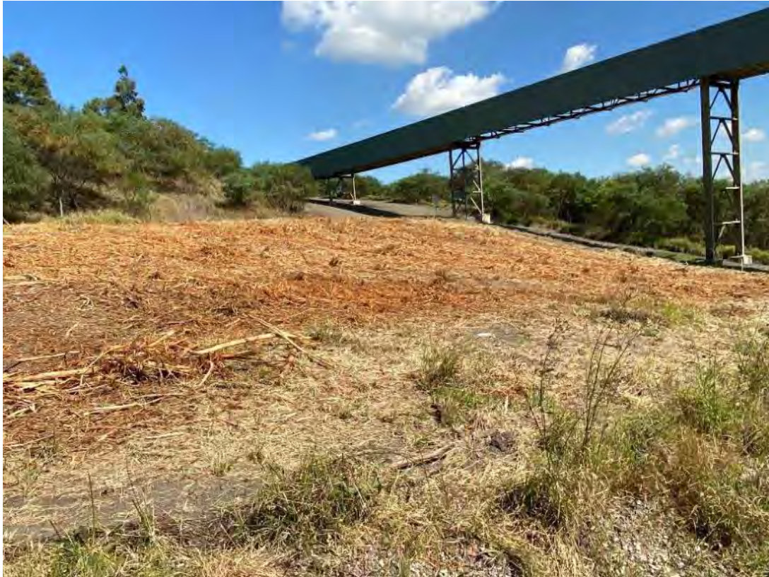
Plate 31 – Evidence of initial marking and mulching for PRP implementation
