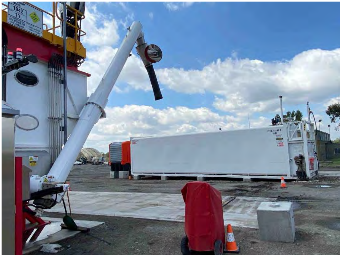
Plate 12 – Ammonium Nitrate Plant
