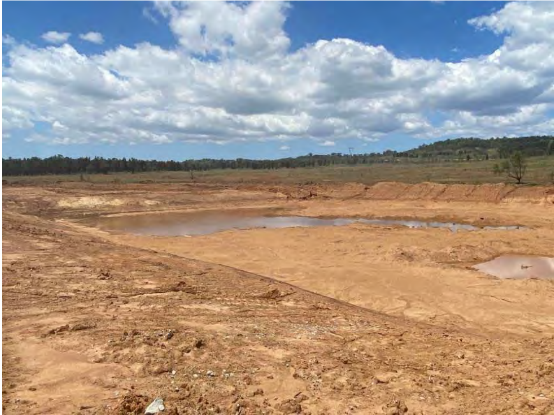
Plate 37 – Mitchell Pit Dam under construction
