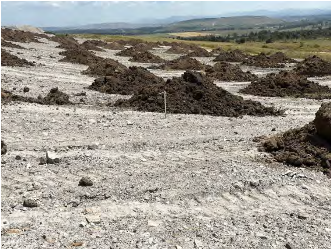
Plate 61 – Active rehabilitation works topsoil spreading on contour banks
