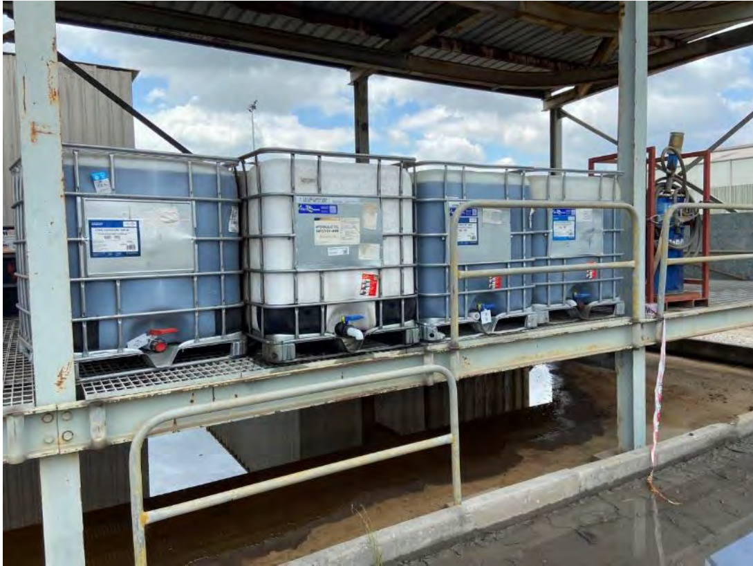
Plate 11 – Permanent bunding structures sufficient with regular cleanout of bunds evident
