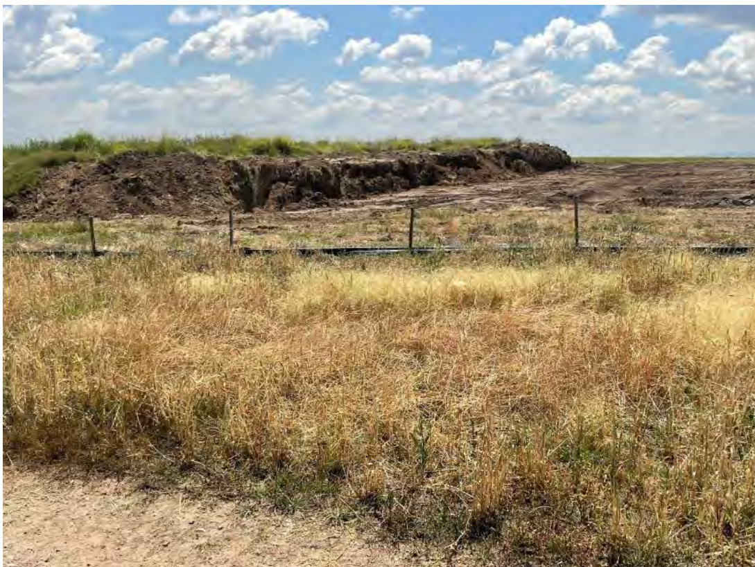
Plate 62 – Sediment and erosion systems in place for topsoil stripping
