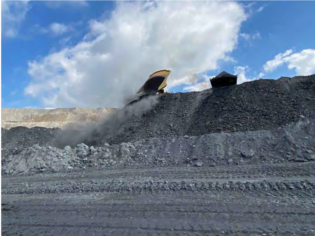
Plate 3 – Trucks dumping overburden with minimal dust production noted
