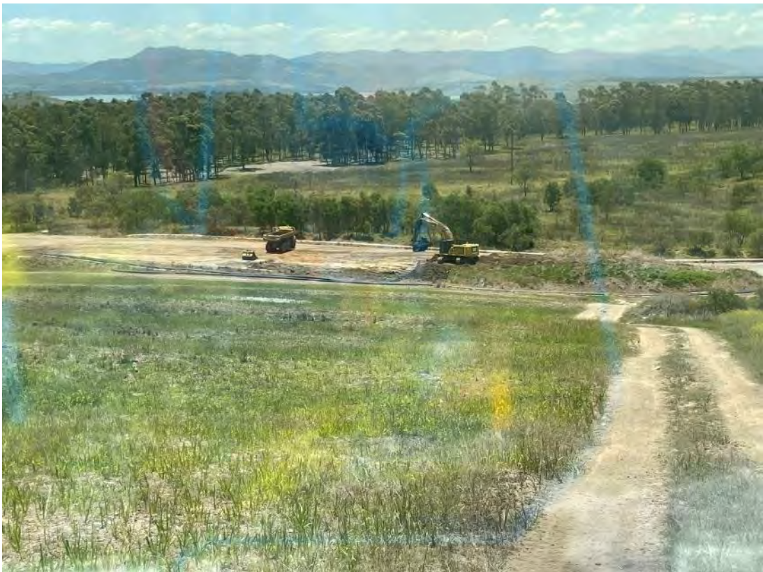
Plate 60 – Active rehabilitation works
