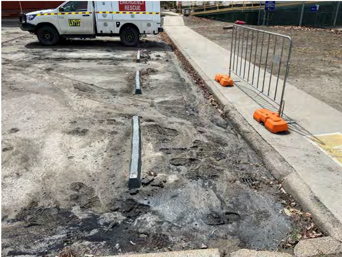
Plate 9 – Sediment build up following rain events in southern muster point carpark area
