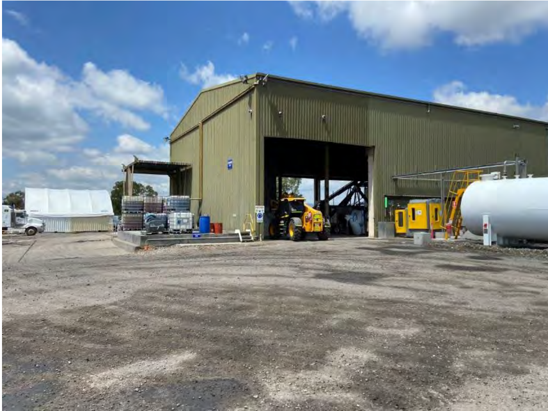
Plate 13 – Ammonium Nitrate Plant
