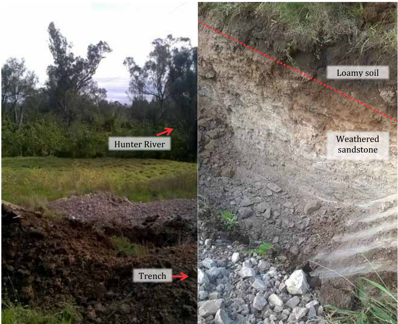
Figure A- 6 Trench location and trench lithology
